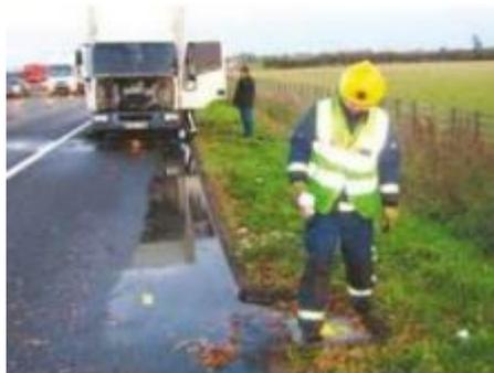
A firefighter contains all on a roadway using a clay drain mat following a vehicle fire.
