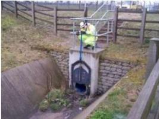
Sluice valve Photo courtesy of Carillion-URS
