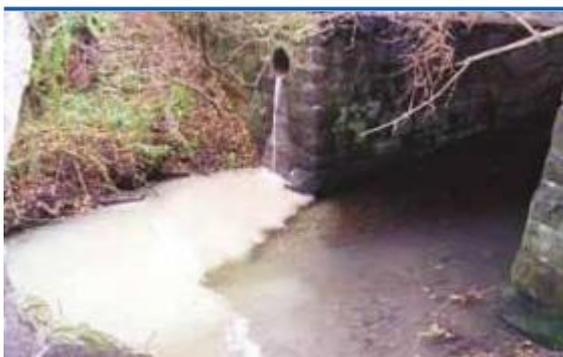
***An example of a pollutant that has travelled through a drainage system to discharge into a nearby river***
