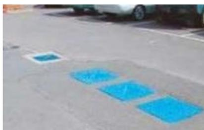
***The older style of oil separator can often be identified by three in-line inspection covers. Where these discharge to surface water, they should be colour-coded blue***
