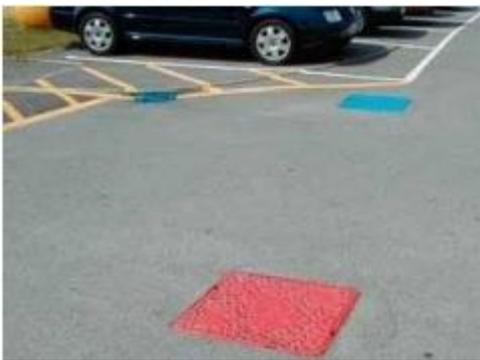
***Drain covers and grills at industrial or commercial premises may be marked with colours, for example red for foul and blue for surface. Other sites may have other types of pipe work such as radioactive water or oily water.***
